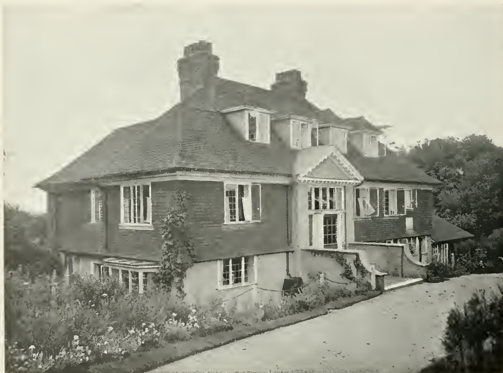
THE ENTRANCE FRONT, HOOKEREL, WOKING, SURREY, A COUNTRY HOUSE BUILT ON THE SOUTH SLOPE OF HOOK HILL. MATERIALS: ROUGHCAST, THE WALLS PARTLY HUNG WITH TILES, THE ROOFING OF SAND-FACED TILES, THE WOODWORK PAINTED WHITE
